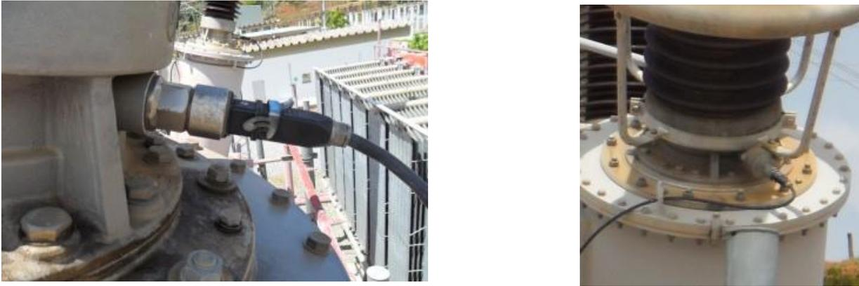
Figure 2 – Example of tap adapter installation. Source: [7].
