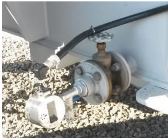
Fig. 07 - Gas and Humidity Monitor
