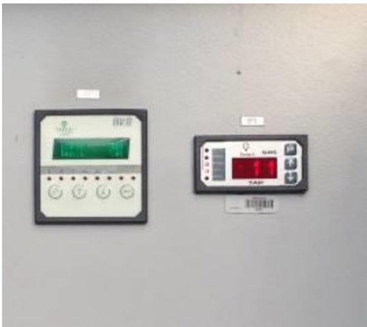
Fig. 06 - Voltage Regulator and Paralleling Supervisor
