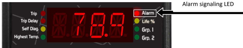
Figure 23 - Alarm signaling LED indication
